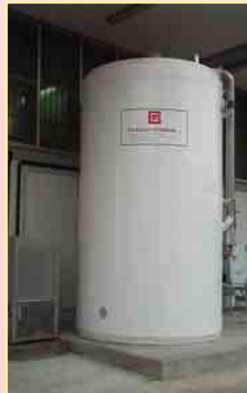
Glass-fibre silos \varnothing 3 meters h 12 meters, 70m 3 capacity installed to a manufacturing firm of carbonated drinks.
