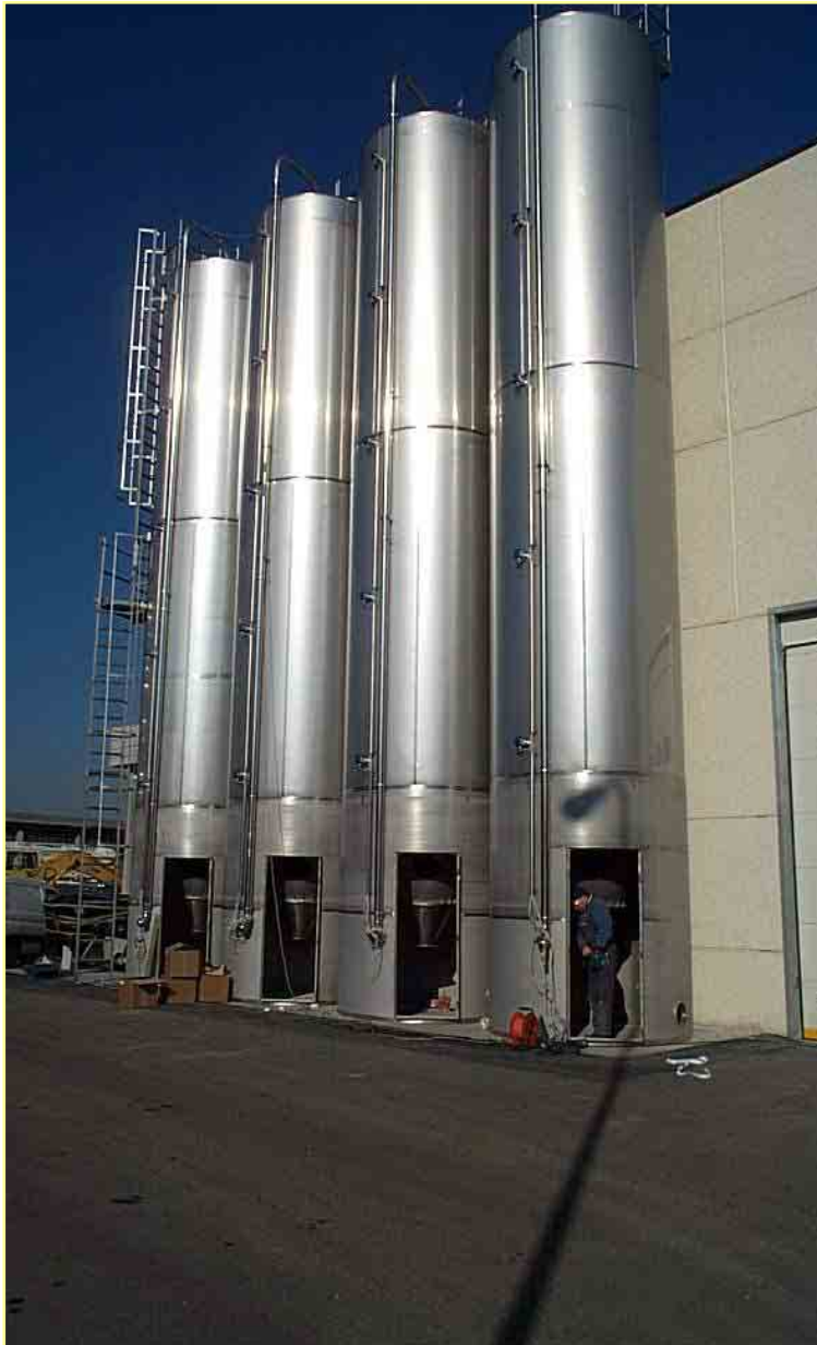
Inox steel AISI304 silos for the storage of 270 quintals of plastic dusts
