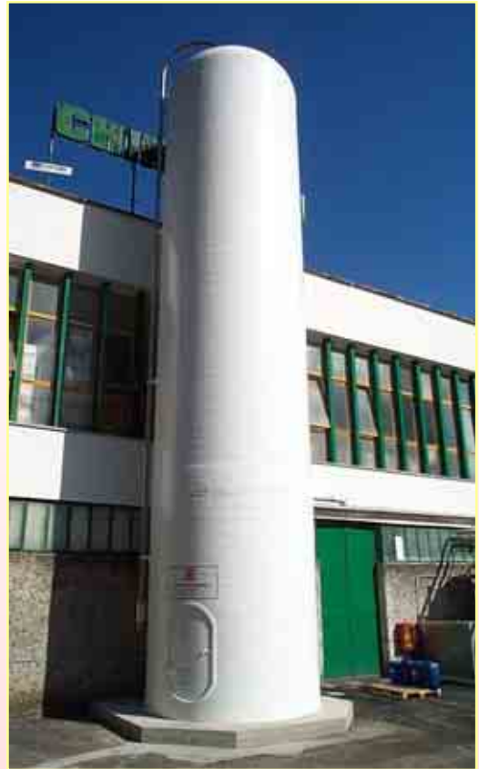
Glass-fibre silos \varnothing 3 meters h 12 meters, 70m 3 capacity installed to a manufacturing firm of carbonated drinks.
